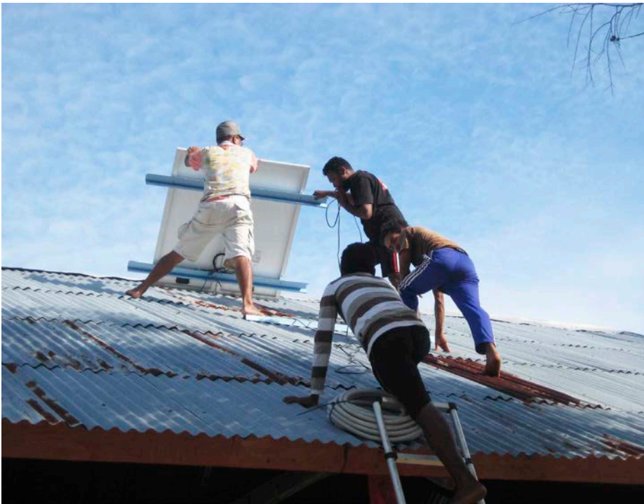
↑ Installing the panels on the school roof.
