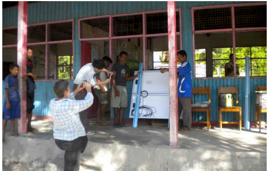
↑ The panels at the Atecru school before installation.
